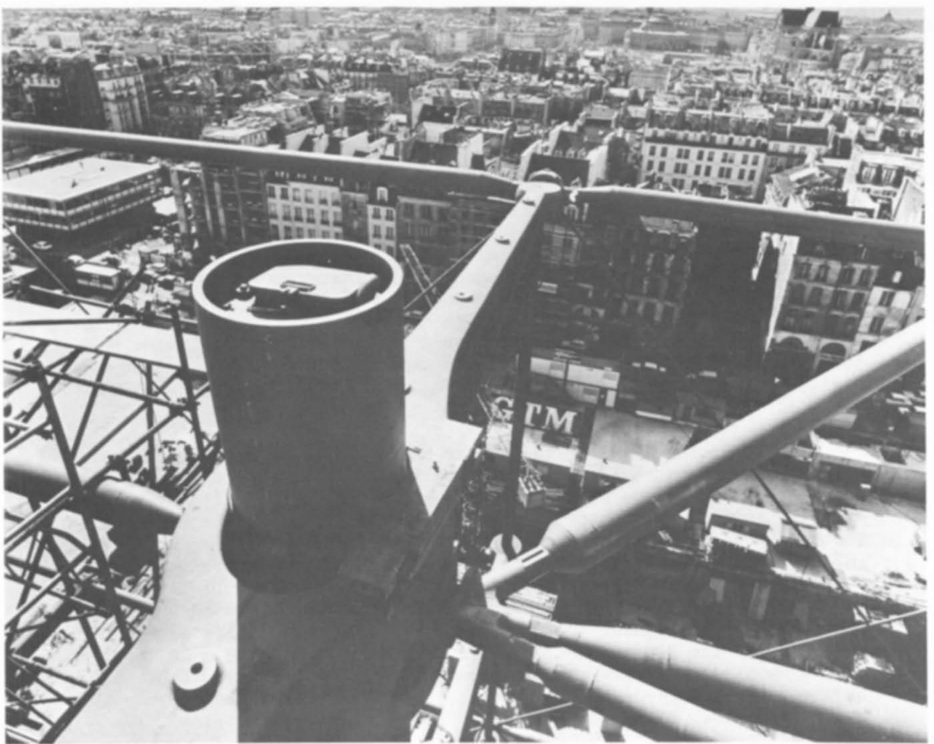
Figure 7—Structure at the top of the Beaubourg Centre in Paris, showing cast steel nodes (Courtesy of Ove Arup and Partners).
