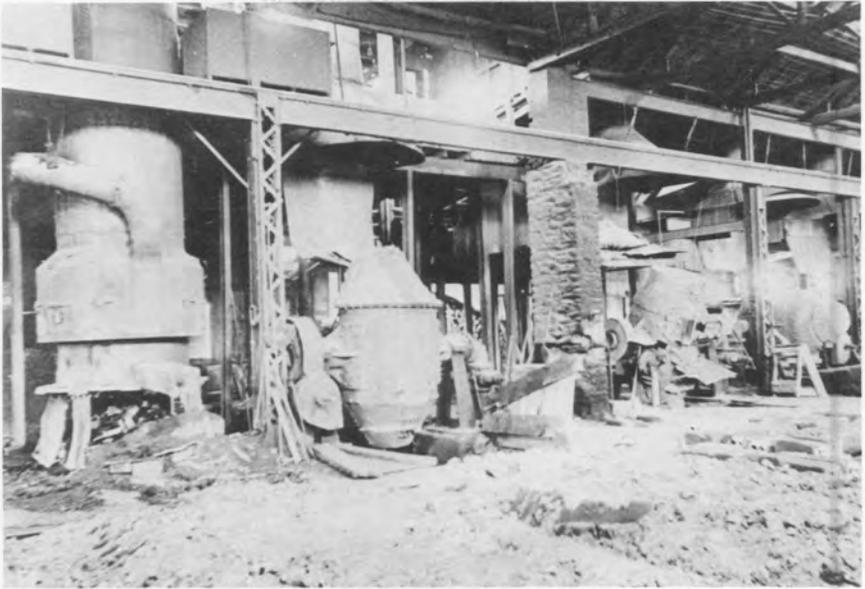
Although the electric furnace was gaining rapid acceptance, the converter still accounted for a greater percentage of steel castings' production. The photo above shows a converter furnace department before starting work. Below, while the metal is removed from one furnace, a second is being blown and a ladle is pre-heated under an oil burner.
