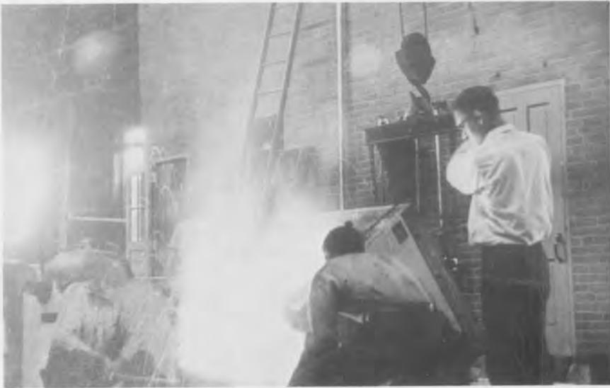
*In contrast to the size of the open-hearth is this small 1/2 ton per hour circular arc electric furnace installed in 1928 by Lebanon Steel Foundry for the production of stainless steel castings.*
