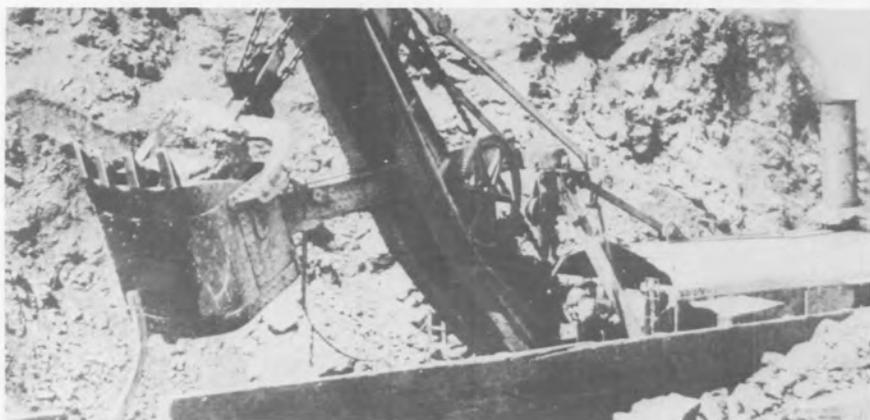
*The construction of the Panama Canal required a wide and dramatic use of steel castings. Buckets for shovels and dredges cut into the mountains and swamps of the Canal Zone.*
