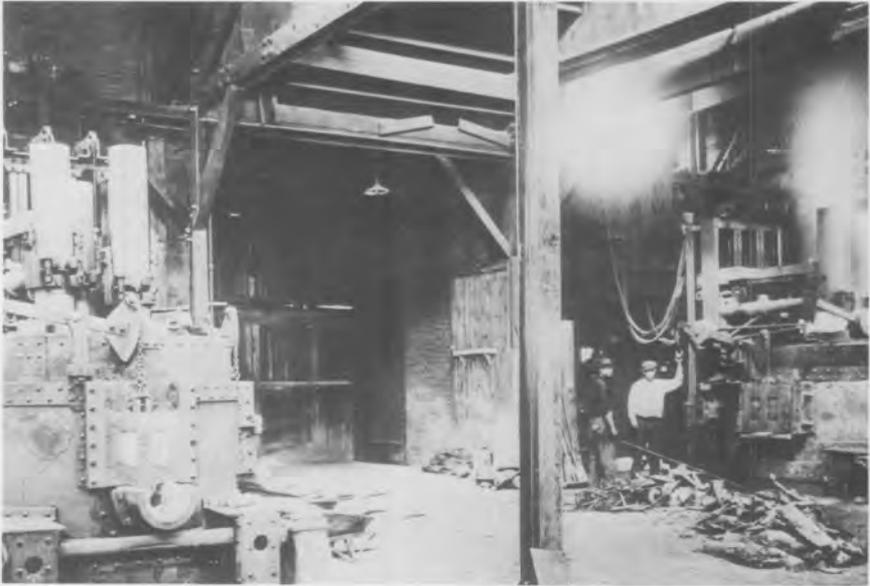
*The electric furnace was gaining rapid acceptance. Pictured here are two 2-ton circular Heroult furnaces. The furnace on the left was installed in 1915, and when its success was proven, the second furnace (on right) was installed.*
