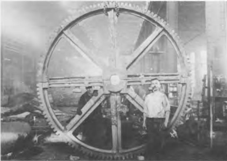
*A scene from the cleaning room shows two chippers and one of Maynard electric's first large gear castings.*
