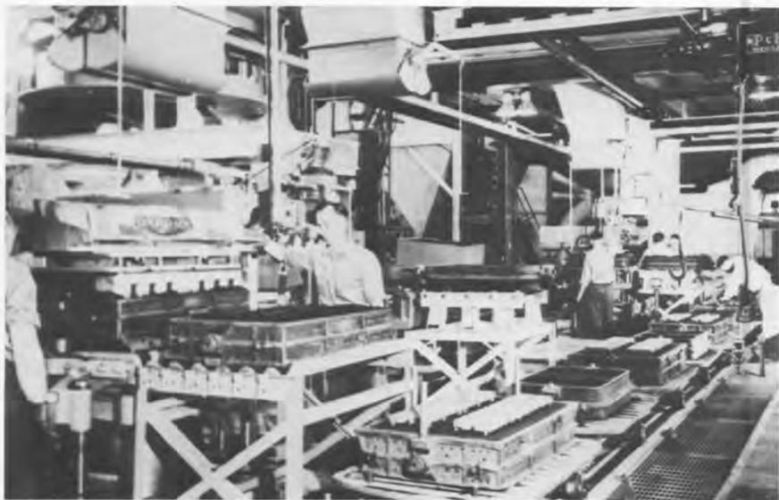
Automation was a watchword of the fifties as foundries strove to increase production and efficiency. This 1956 photo shows molding machines and mold conveyors in the G.M. Development Center.
