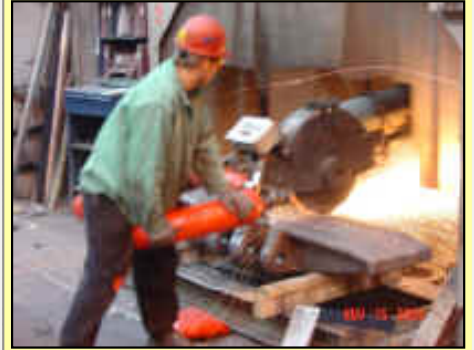
Swing Grinding the Riser Stubs
