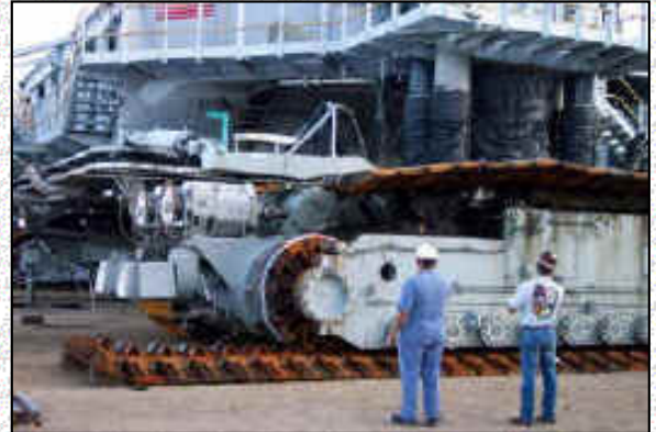
Track Belt Being Installed on the Transporter
