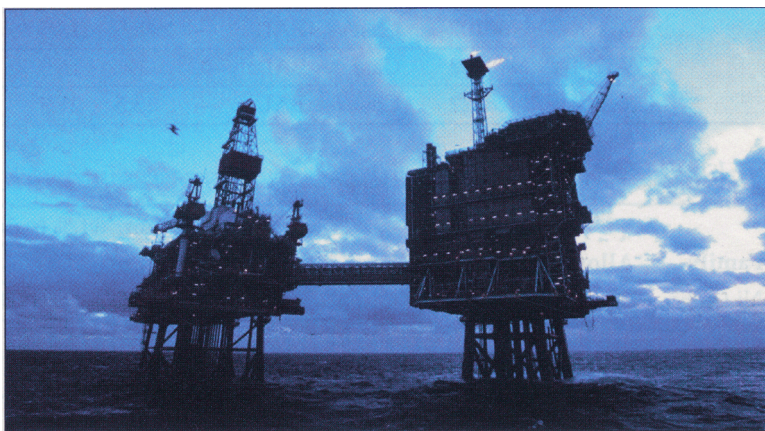
Offshore oil rig structures must be built of alloys that resist seawater corrosion. Image courtesy Rolls Royce.
