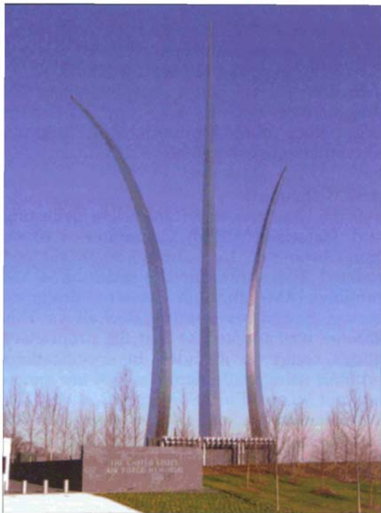
The Air Force Memorial in Washington, D.C., ranks as one of the world's largest structural applications of stainless steel. It consists of three stainless steel spires reaching 64 m into the sky. Each spire has a 19-mm-thick skin of 531600 stainless steel covering a core of reinforced concrete. Image © 2008, Jon Rochetti, www.TheDCTraveler.com.
