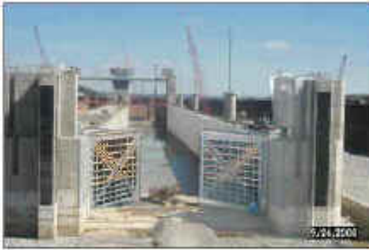
Gates under Construction
