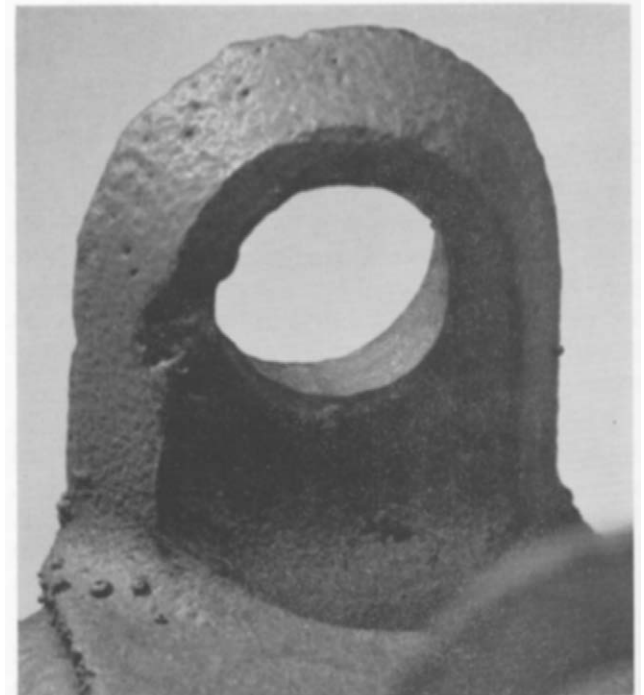
Figure 3—Slag inclusions in cored hole area.
