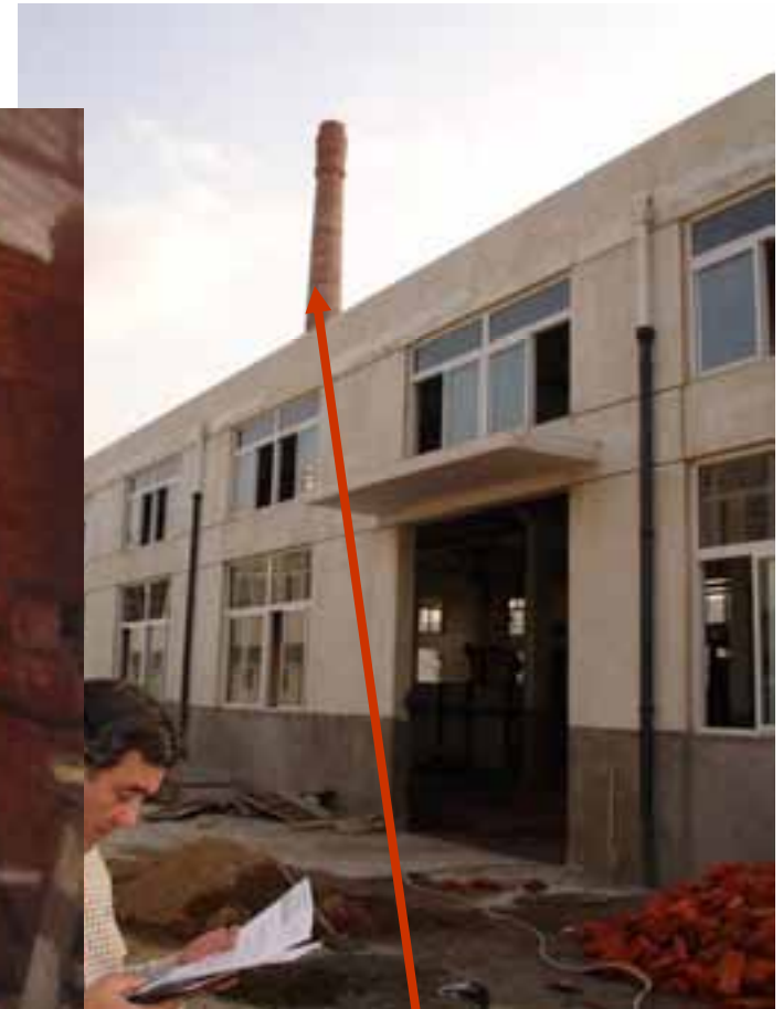
Chimney for spent wax
